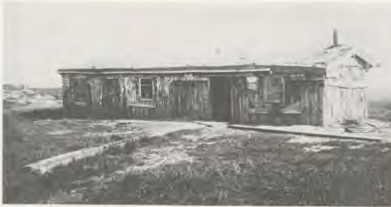
This was one of the very first structures in Richardton. It belonged to Jim Reilly and was located just southwest of the present water tower. Reilly, the grandfather of Fr. James Reilly of Assumption Abbey, worked for the NP Railway as a water pumper. The shanty is made of railroad ties.
